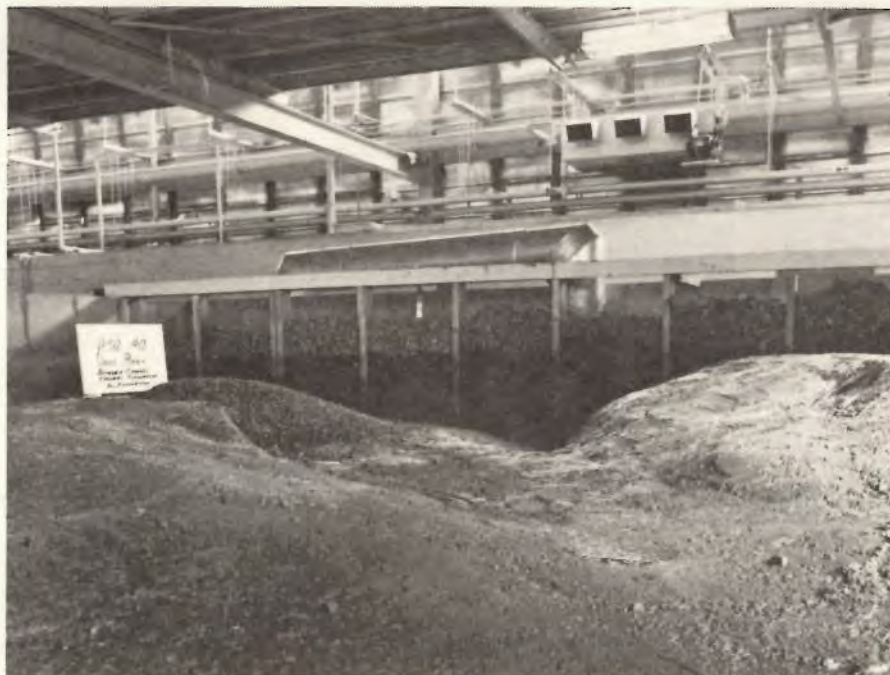
Figure 7.—Approach channel with proposed excavation filled in, located about 500 m upstream of spillway crest. P801-D-79579.
