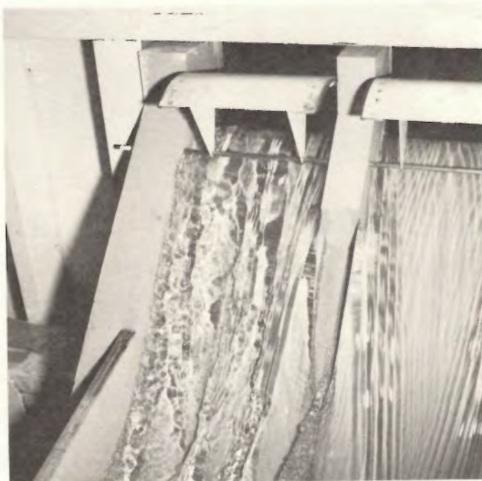
Figure 10.—Impingement of flow on the gate trunnions: Q = 2600 \text{ m}^3/\text{s} . P801-D-79582.
