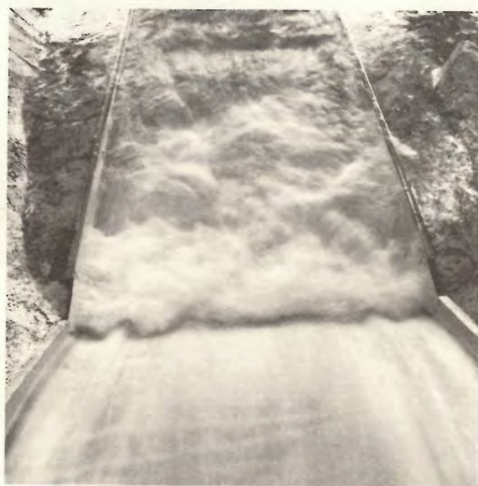
Figure 24.—Spillway stilling basin operation for Q = 2000 \text{ m}^3/\text{s} and tailwater EL 33.4. P801-D-79589.
