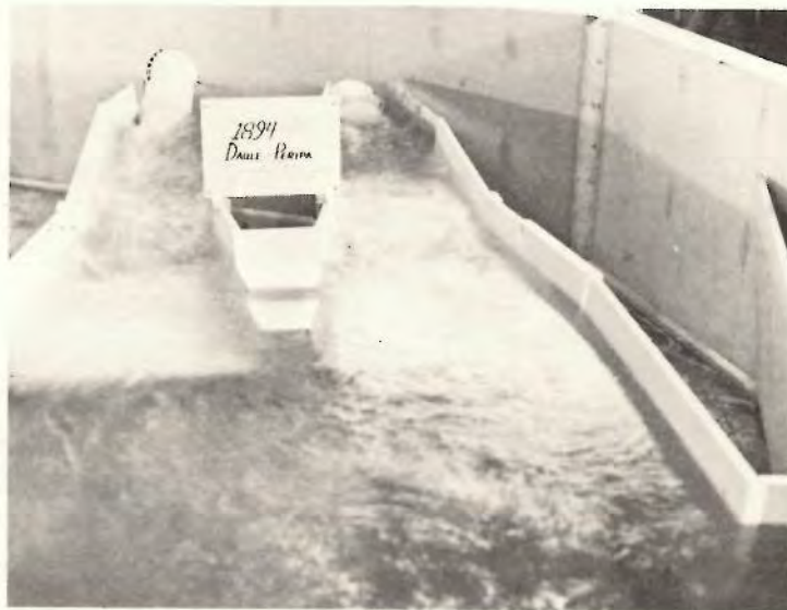
Figure 42.—Diversion stilling basin operation, reservoir EL 40, Q = 1472.7 \text{ m}^3/\text{s} , tailwater EL 30.3. P801-D-79600.
